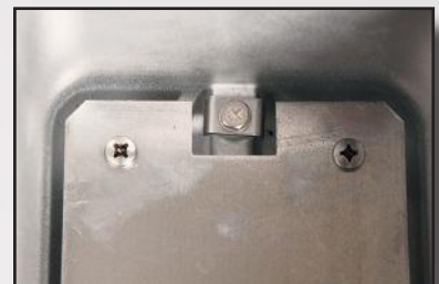
Internal earth screw in body
